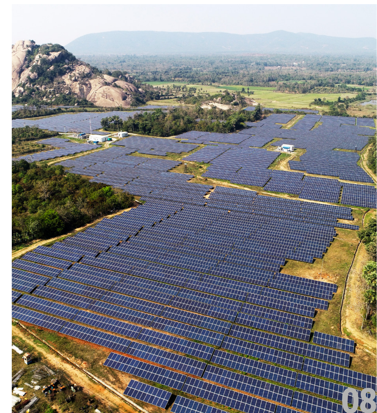
📷 Vizianagaram Solar Power Plant
