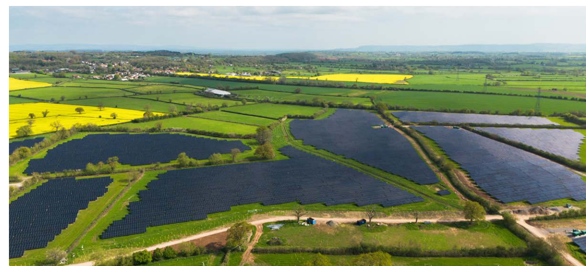
📷 Larks Green solar PV project in South Gloucestershire, UK.
